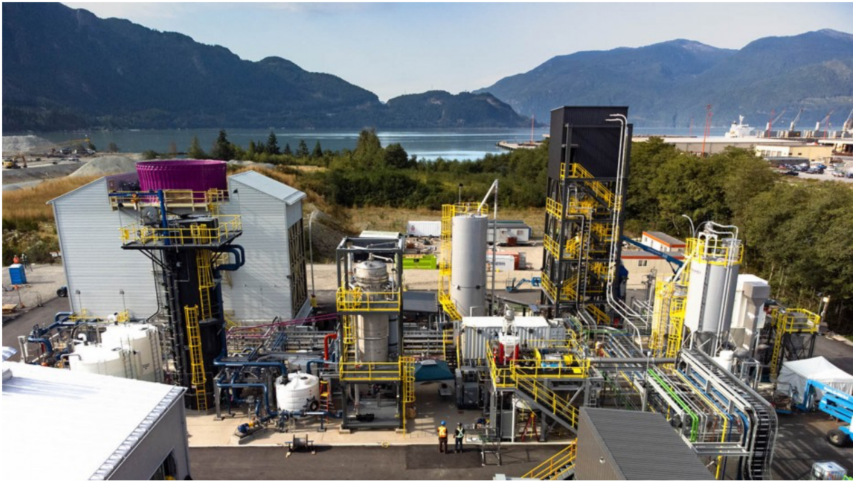
Carbon Engineering Innovation Centre in Squamish
