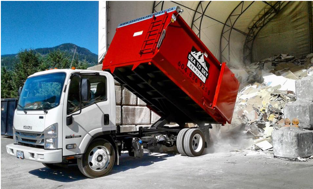
Drywall being dropped off at New West Gypsum Recycling. 40 years ago, this waste would have gone to a Vancouver landfill. In California, much of it still does.
